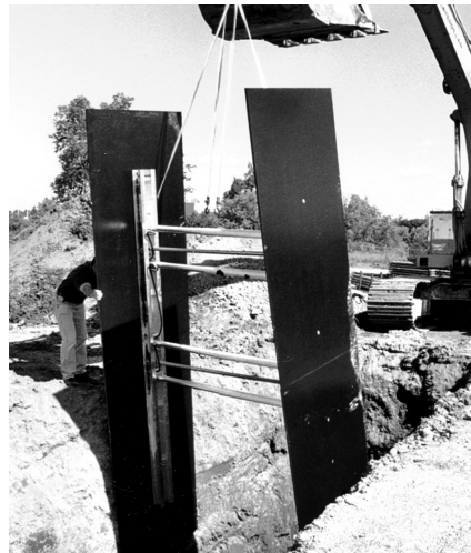
Rails may be bolted to Finform, etc. (See pg. 1 for alternate sheeting)
