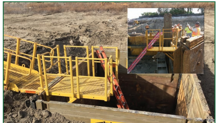
The internal ladder platform cage is designed to extend beyond internal walers on ClearSpan configured Slide Rail Systems, providing quick-access to the bottom of the shored excavation.
