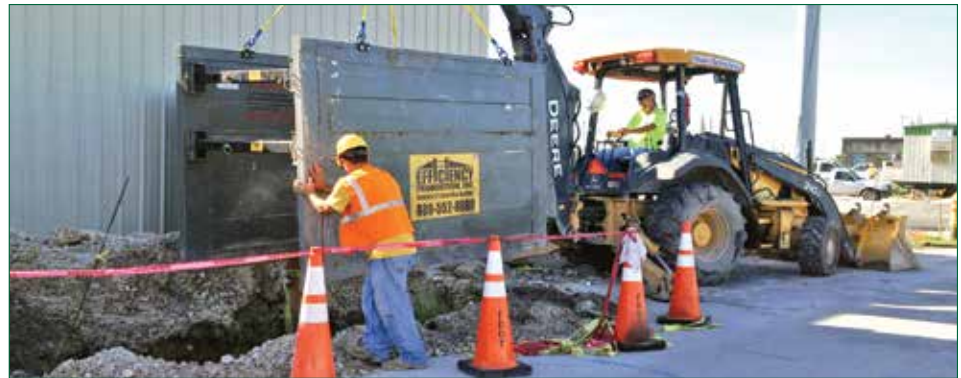
XLAP-SF 75 mm Aluminum steel frame double Sidewall Trench Shield
