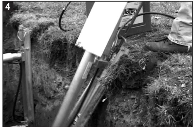
4 The shore will fold as it is pulled out. Remove tools, fold shore flat, and carry to the next installation spot.
