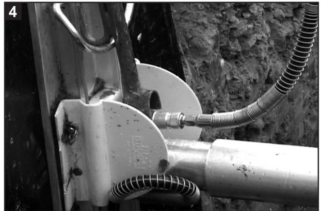
4 To remove the hose, place the release tool flange behind the collar of the quick disconnect fitting. The hook will be toward you. Pull the tool toward yourself, using the hook as a pivot, the hose will come off. After hose is disconnected, clip hose to the top of pump. Open valve on pump and move to the next shore.
